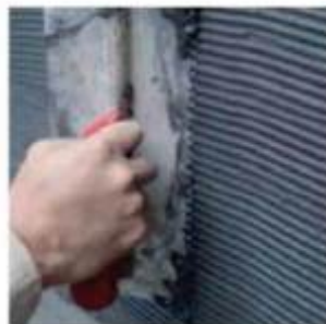
2. Scrape off the cement slurry on the wall
