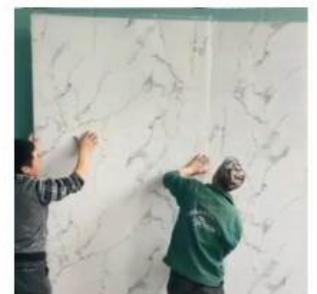
3. Install directly on the wall.
